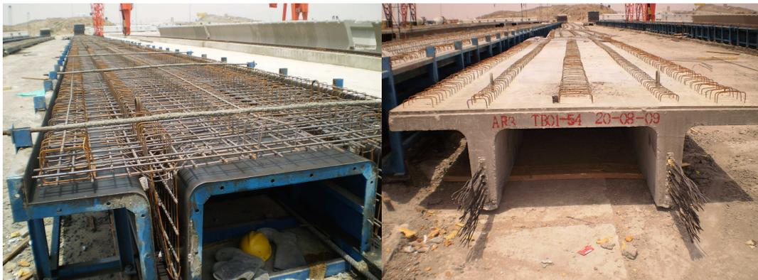
Figure 30: Double Tee construction
