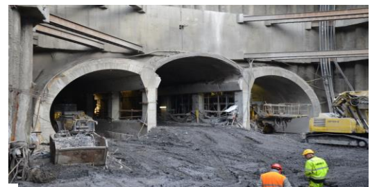
Figure 30 : Construction de la station
